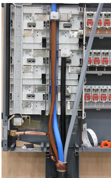
Routing of the Grey conductor:
