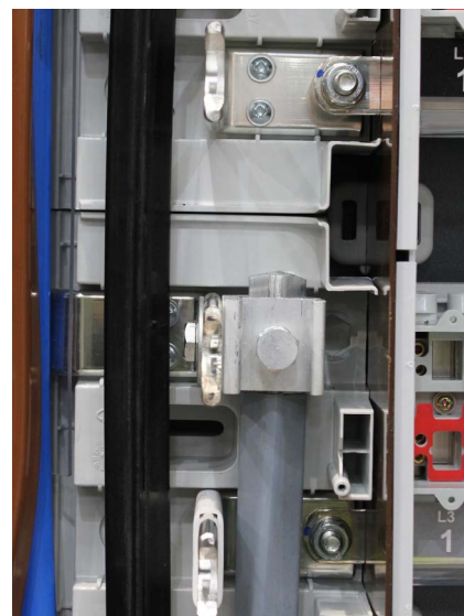
Making Off the Grey conductor:
