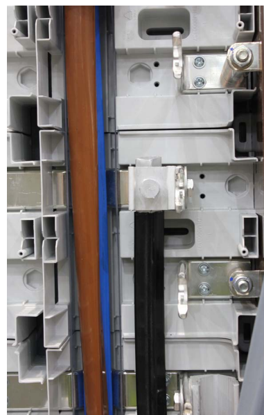
Making Off the Grey conductor:
