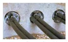
**RDSS Rayflate inflatable** duct seal
