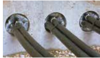
RDSS Rayplate inflatable duct seal
