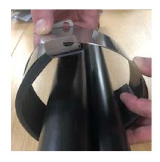
1. Wrap liner around cables to determine length. Discard excess liner.
