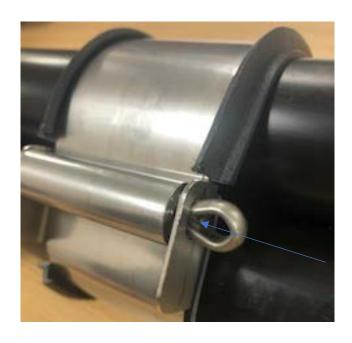
6. Once cleat is secure and tight around cable, hammer pin into the slot so that it is fixed and unable to move.
