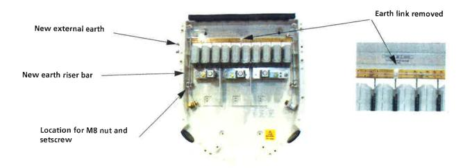
3. Reposition the brass BTCNE in its new position on the earth bar and tighten to a torque setting of 22Nm. Install the aluminium neutral connector provided in the kit on the neutral bar in the position shown and also tighten to a torque setting of 22Nm.
